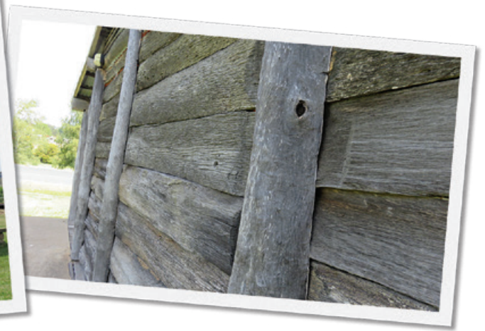
Exterior wall of the slab hut
