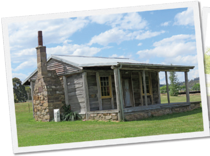
All Saints' School: the original slab hut
