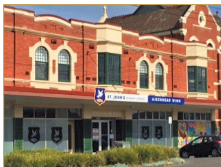
The Aikenhead Wing at St John the Baptist Catholic Primary School, Clifton Hill, Victoria
