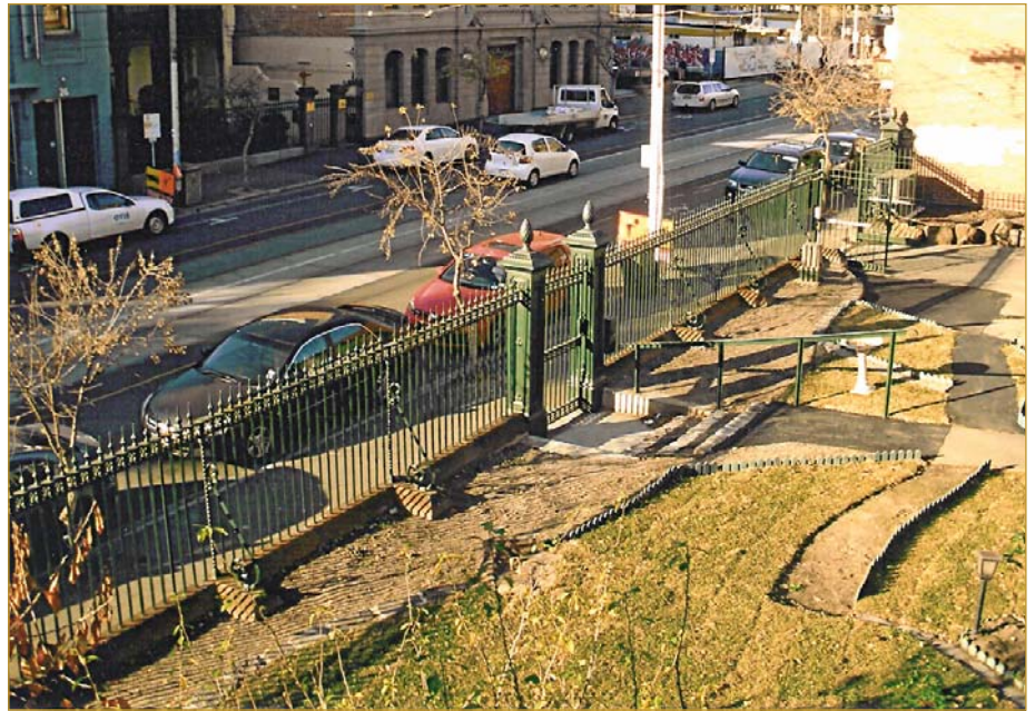
The newly restored fence at last! Garden beds ready for plantings. Photo courtesy Bernadette Culhane rsc
