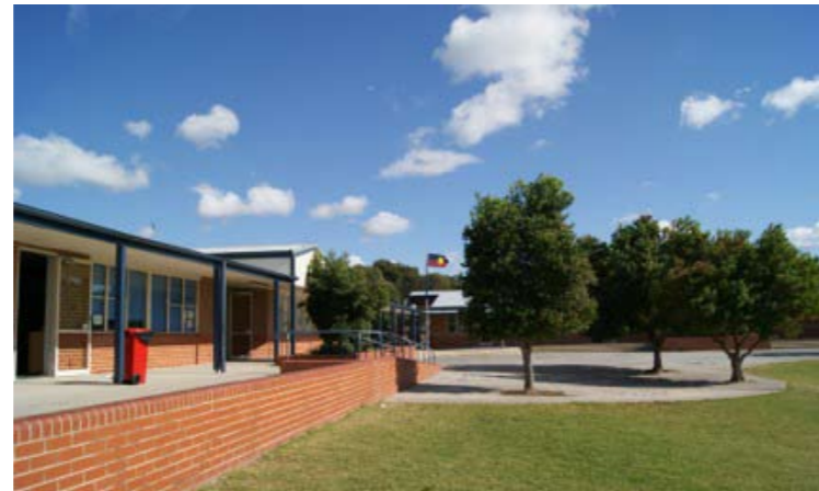
Nazareth Catholic Primary School, Shellharbour City
